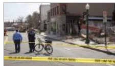
Mamaroneck building collapses
